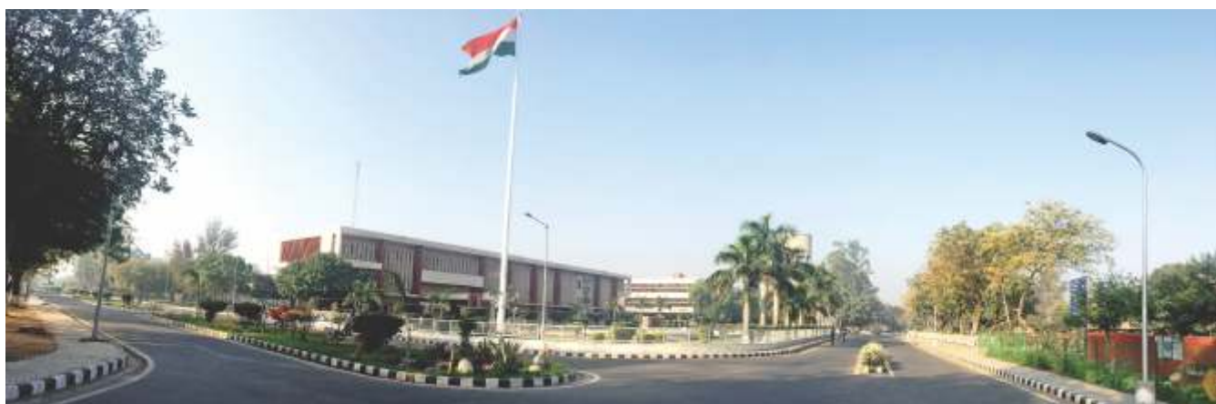
Administrative Block CCSHAU, Hisar
